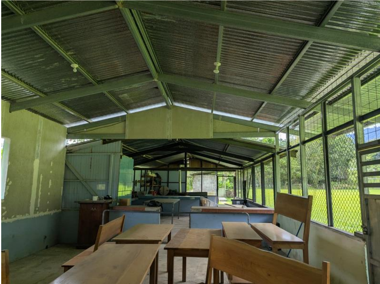
Existing covered infrastructure provides a serviceable asset base for rehabilitation, maintenance and future capacity planning.
